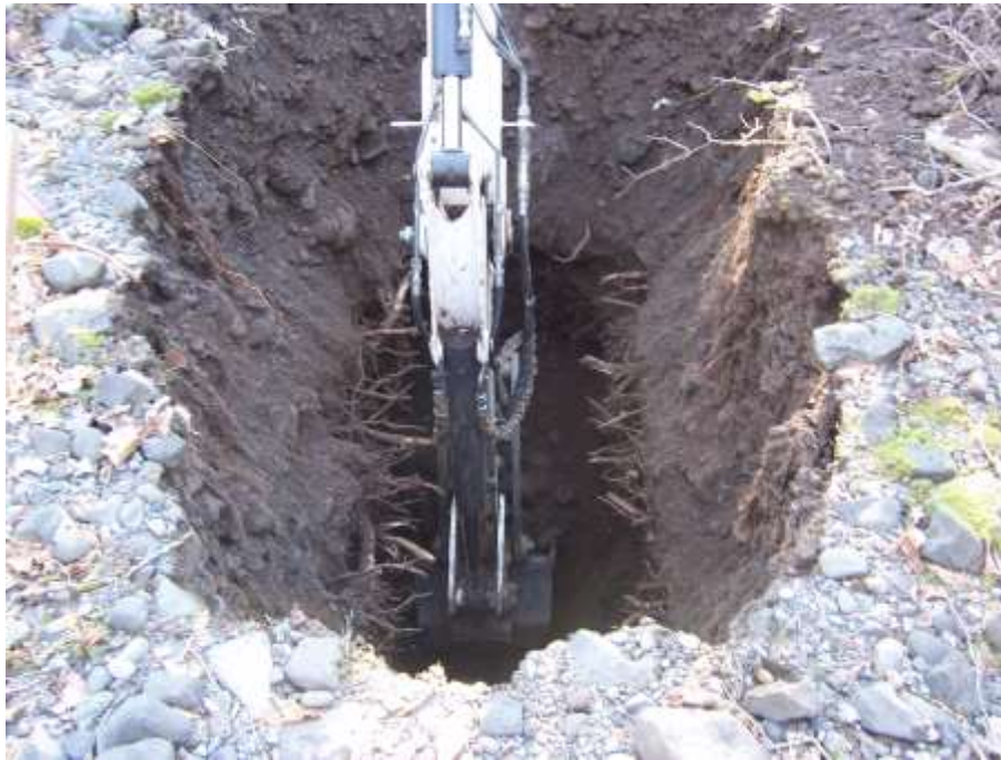
Figure 21. Excavation (typical) 8 to 10 Feet below Ground Surface.
