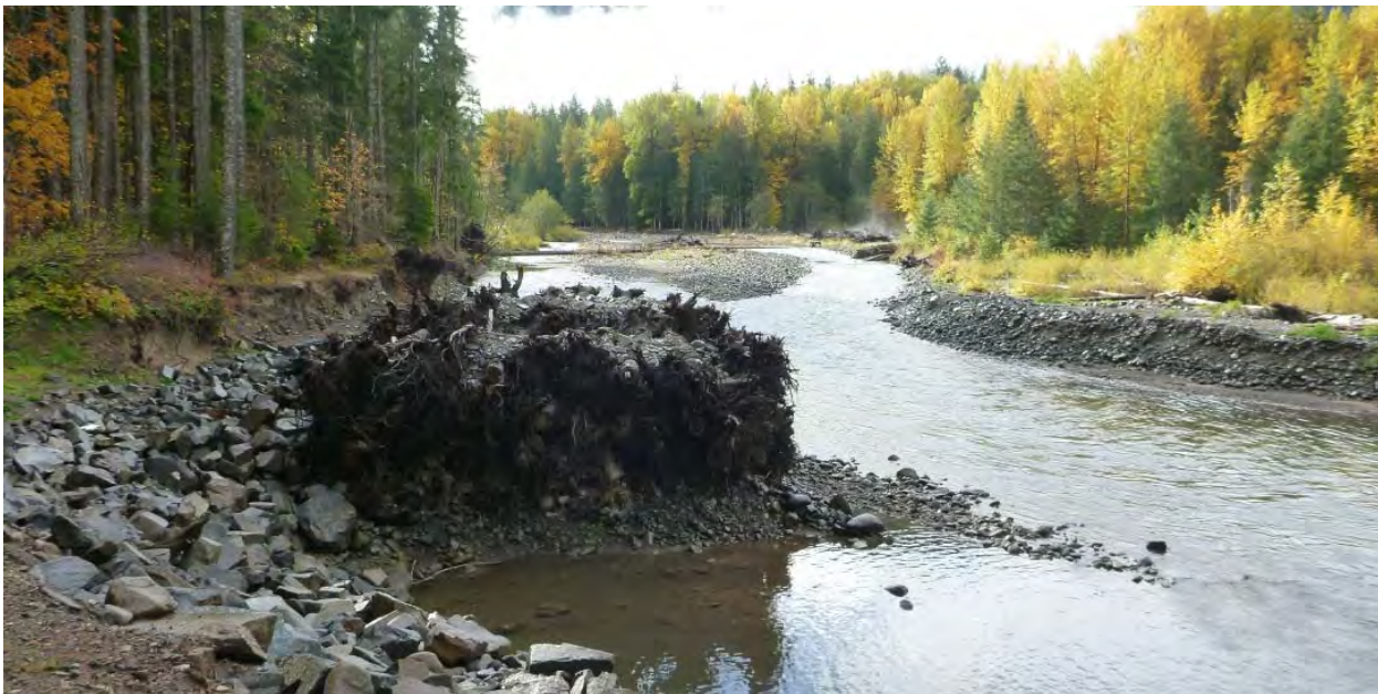
Figure 10. Large engineered log jam at upstream of FS Road 23 repair near RM 21.
