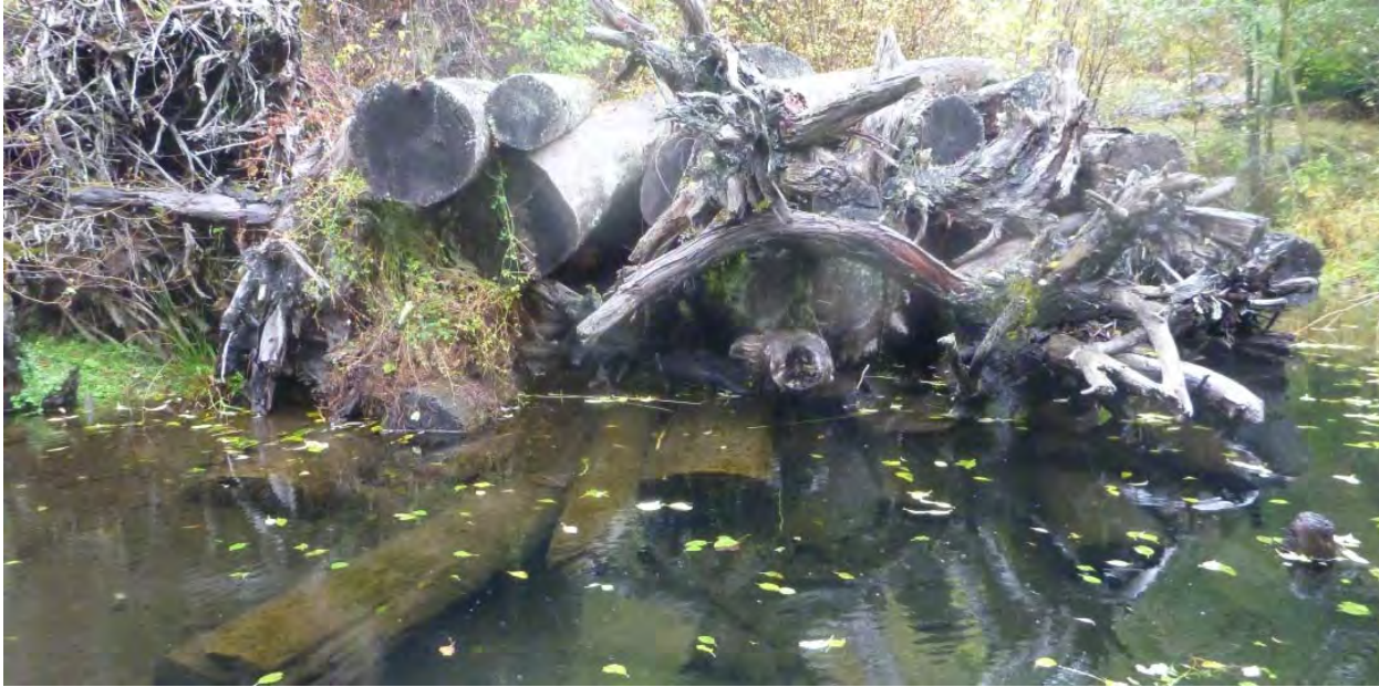
Figure 11. Older engineered log jam placed along FS Road 23 near RM 19 (now in abandoned oxbow).
