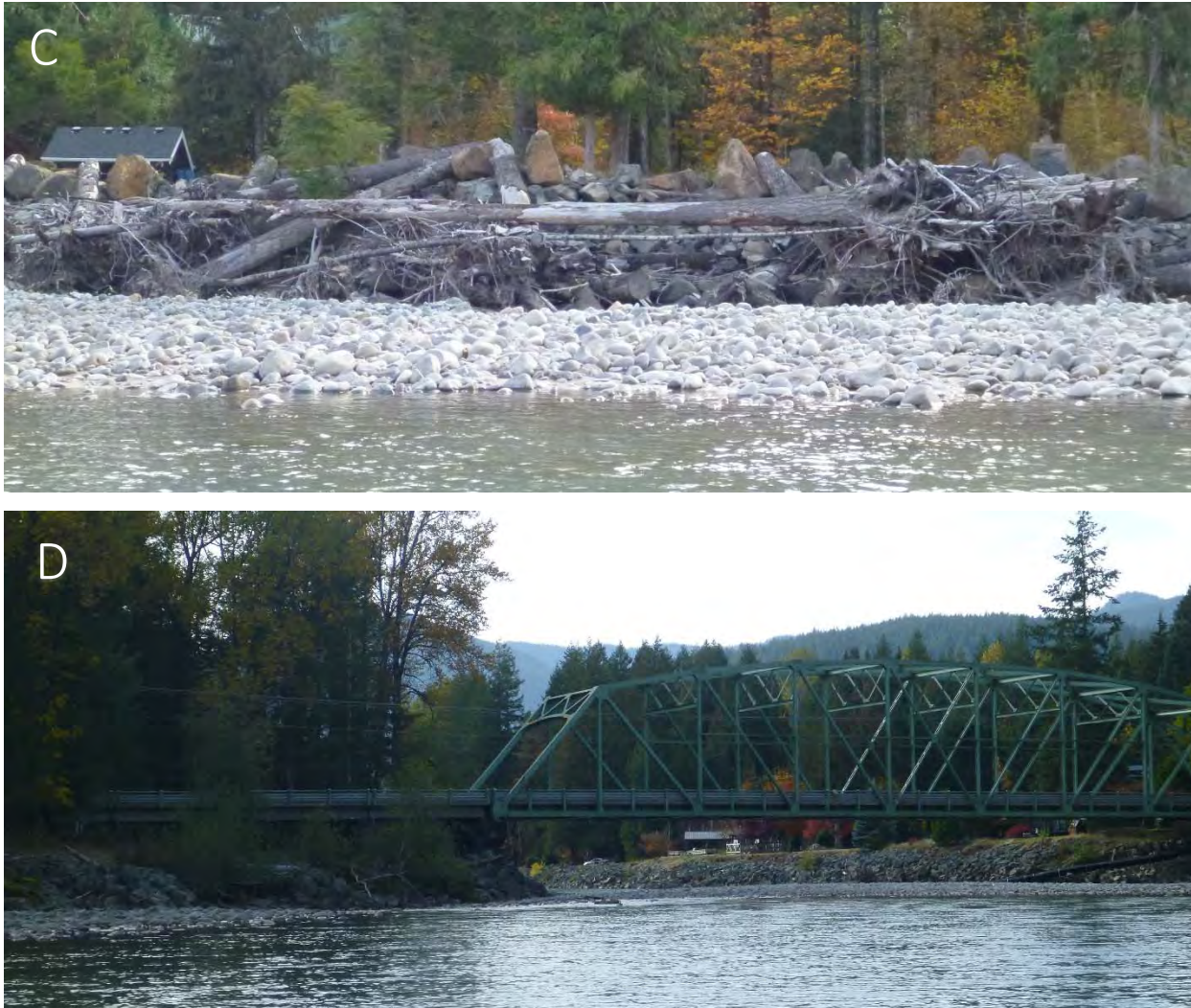
Figure 4. Representative images from the Cowlitz-Packwood LU. A = typical broad flat gravel and cobble bar. B = houses high on south bluff in Packwood area. C = Riprap and large wood bank protection structure on south bank upstream of Skate Creek Bridge. D = Skate Creek Bridge and riprap extending up- and downstream.
