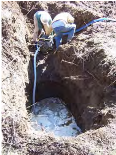
Figure D1. Test Pit 1 Excavation
