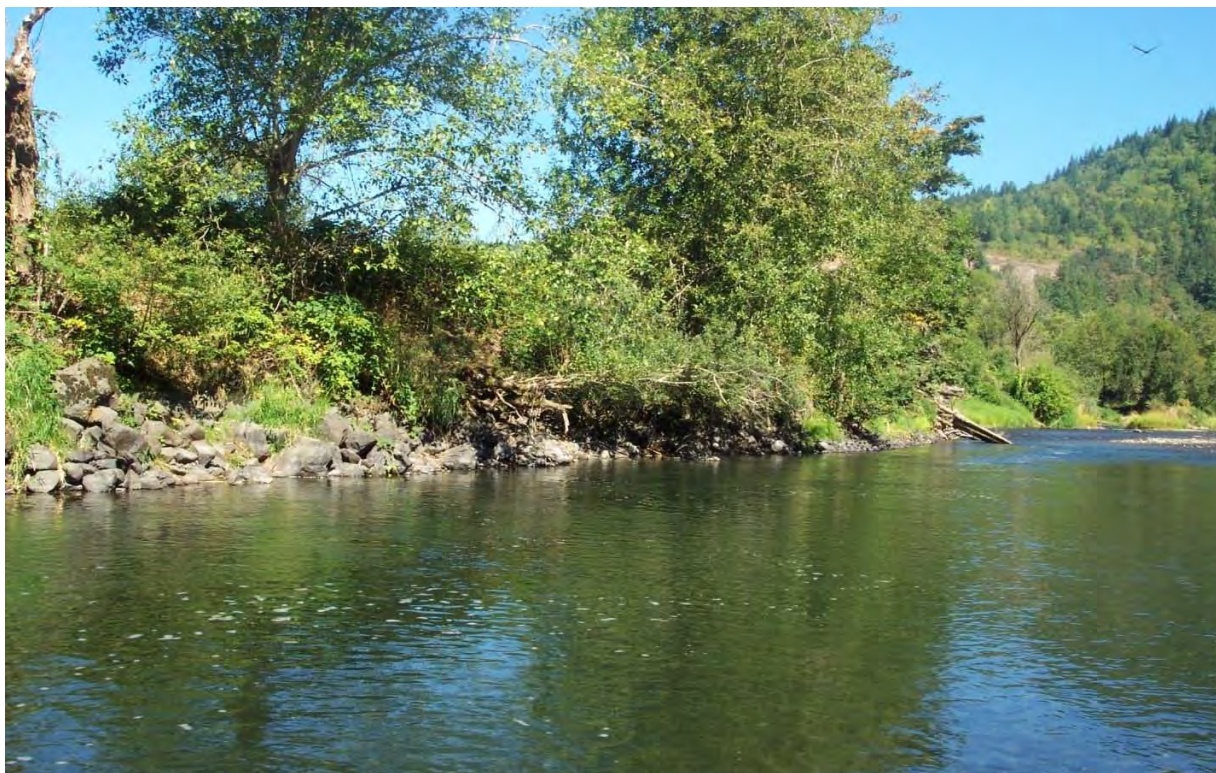
Figure 9. Rip rap along banks of Kalama 2A
