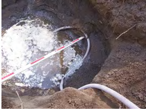
Figure D6. Test Pit 4 Bottom of Hole
