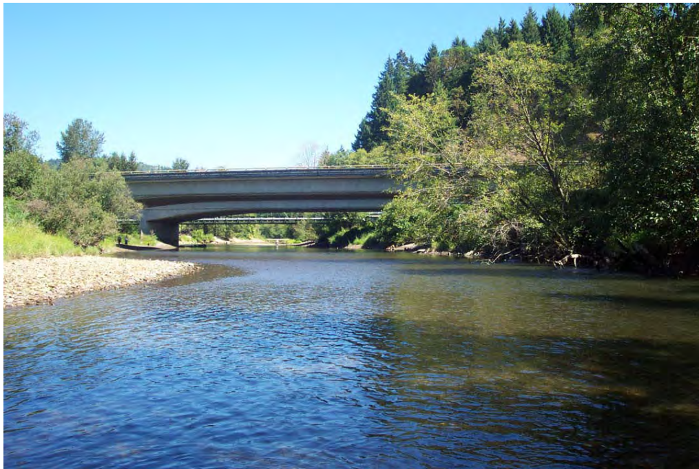
Photo 10 – Upstream view I5 Bridge.
