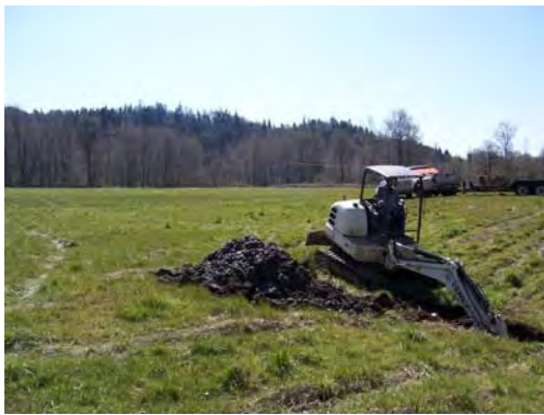
Figure D3. Test Pit 2 Excavation
