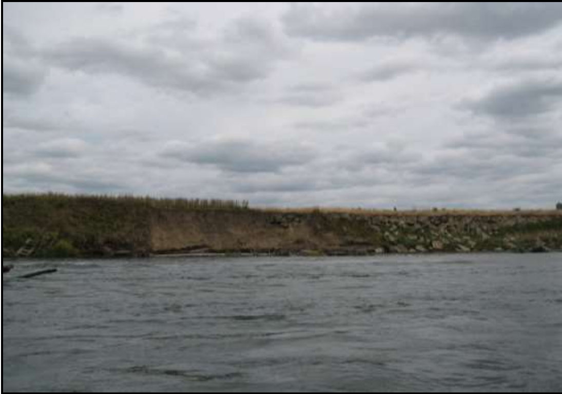
Image looking at left bank near RM 26.0
